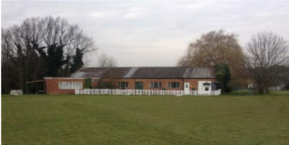
Existing pavilion looking north west (front)
